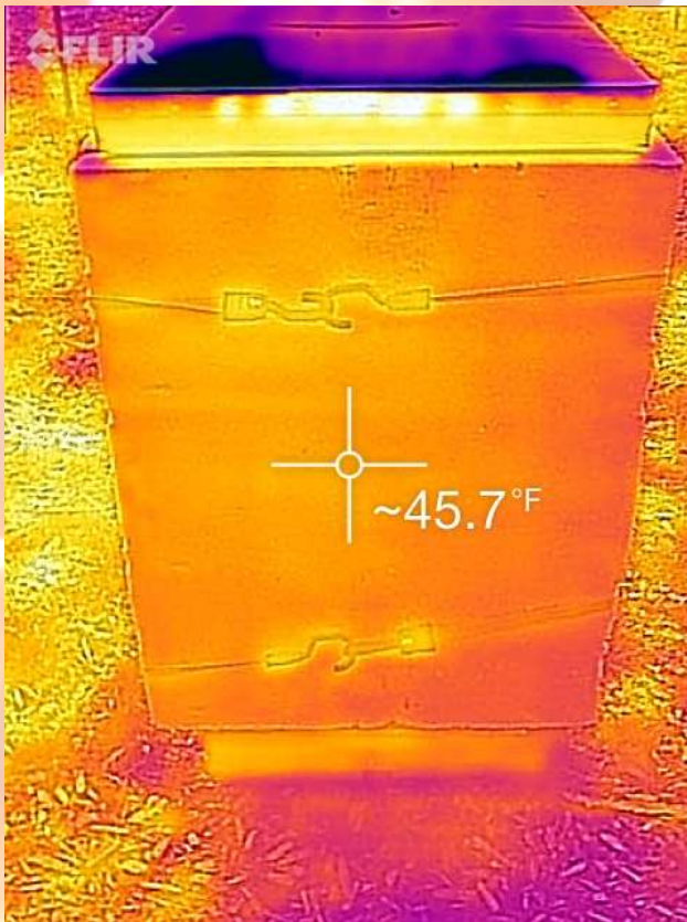
Insulation In Place
